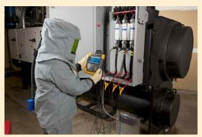
Simply hookup the voltage measurement leads and flexible current probes to the service supplying the motor
